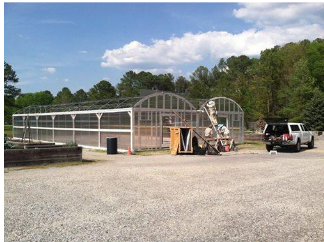
Greenhouse construction last month at Cane Creek
