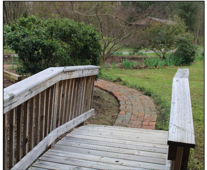
View from the bridge at Cane Creek (bridge built by Cane Creek Crew)
