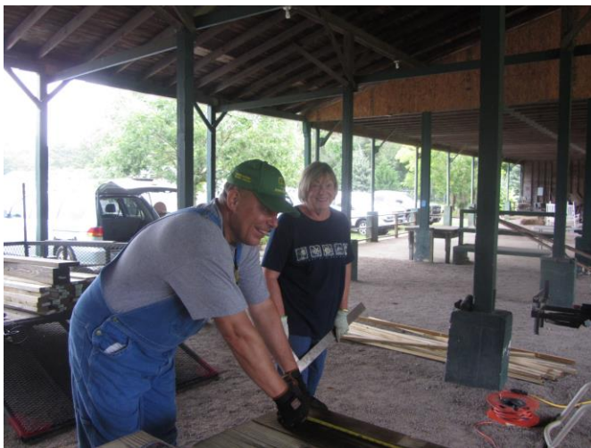
Skeeter Sims and Judy Shew work on ramp
