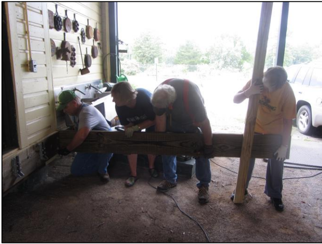
Putting together the Cane Creek wheelchair ramp
